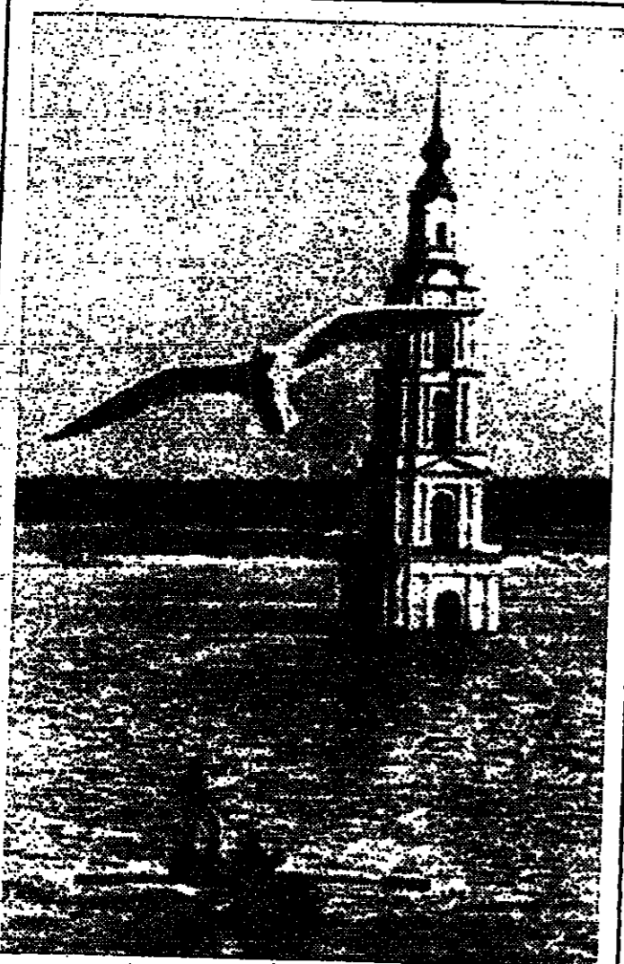
WATER TOWER—Some 30 years ago a dam was constructed near the Russian city of Uglich, on the Volga. A large part of the city was thus destroyed and the area became a huge water reservoir. The tower of the town church, however, is still visible and dominates the entire area like a lonely lighthouse.
